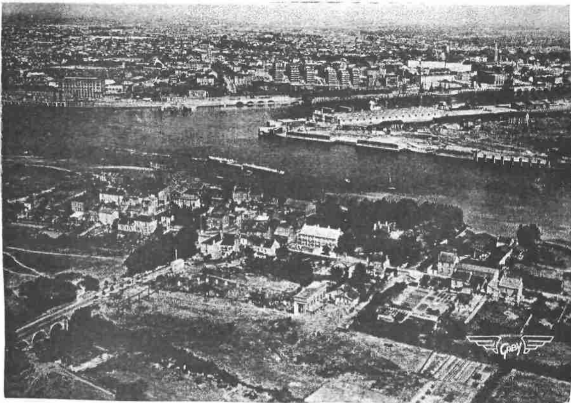
PONT ROUSSEAU (L. INF.) NORTHOUSE - VUE AERIENNE
